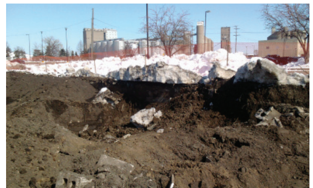
Undocumented buried foundation at U of M job site
