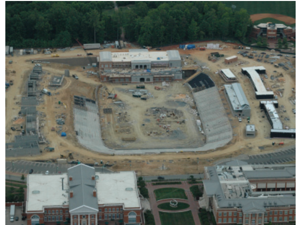
UNCC Football Stadium (progress)
