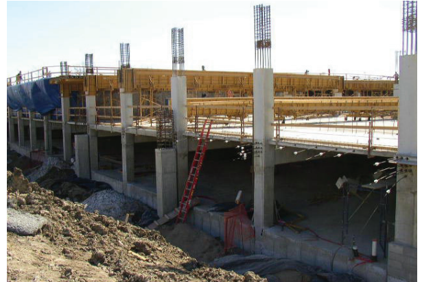
Mystic Lake Parking Structure
