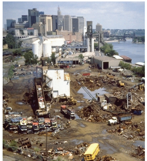
Saint Paul's Upper Landing (before)
