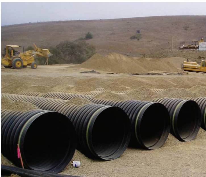
Cambria School Stormwater Storage
