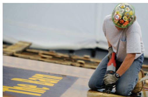
Renovation of Williams Arena by PCL
