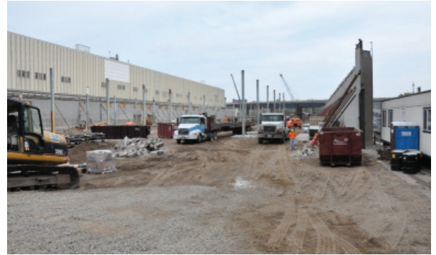
CCLRT O&M Facility
