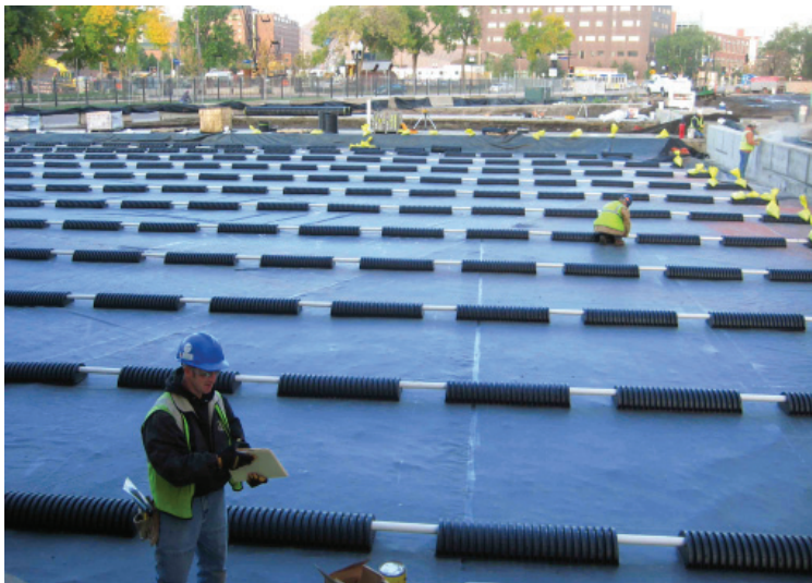
TCF Stadium installation of EPIC system
