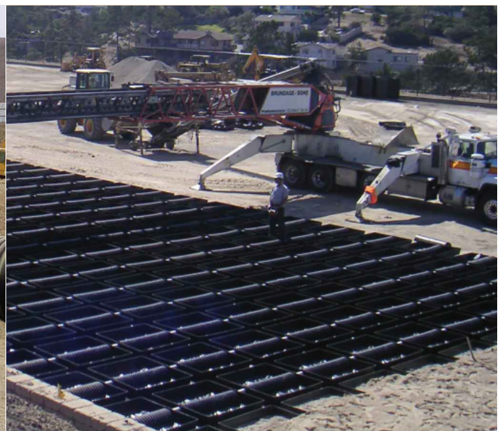
Cambria School Stormwater Storage & Irrigation Installation
